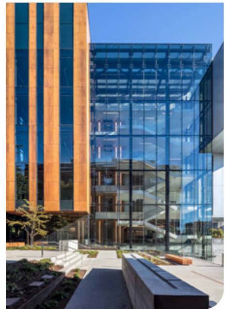
The façade’s point-supported glass system with extra-large Solarban® 72 Starphire® glass panels help fulfill the University’s desire for daylighting, views and transparency.
