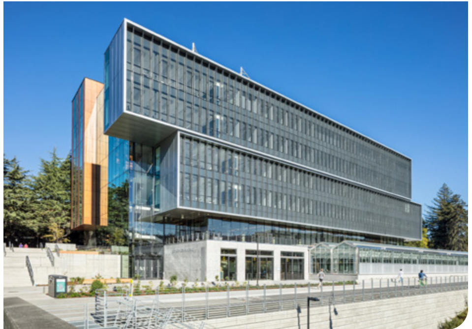
Seattle's University of Washington Life Sciences Building, a 2021 American Institute of Architects' (AIA) Committee on the Environment (COTE) Top Ten winner, features photovoltaic PV fins with Solarban® 72 Starphire® glass on the southwest façade.
